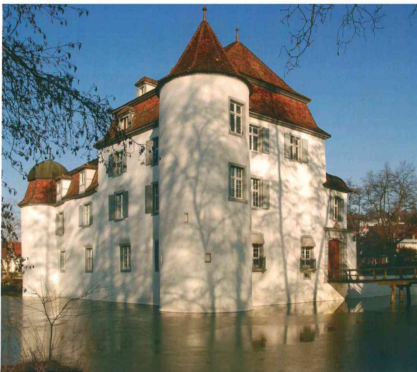
Weiherschloss Bottmingen aus dem 14. Jahrhundert: Heute das ideale Ambiente für ein gediegenes Restaurant. Bottmingen Castle, built in the 14th century, with its distinctive moat – today it also features an excellent and popular restaurant.
